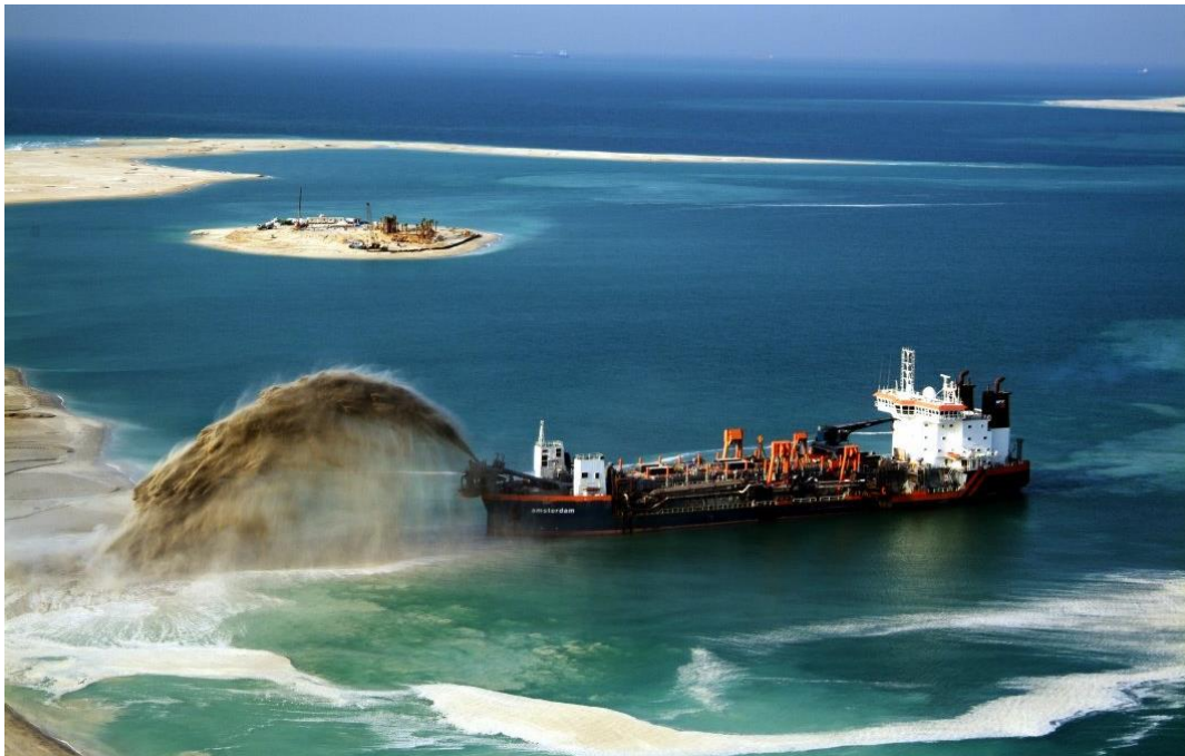
Figure 6: Example of trailing suction hopper dredger placing sediment using “rainbowing” in Dubai (Van Oord, 2005)
