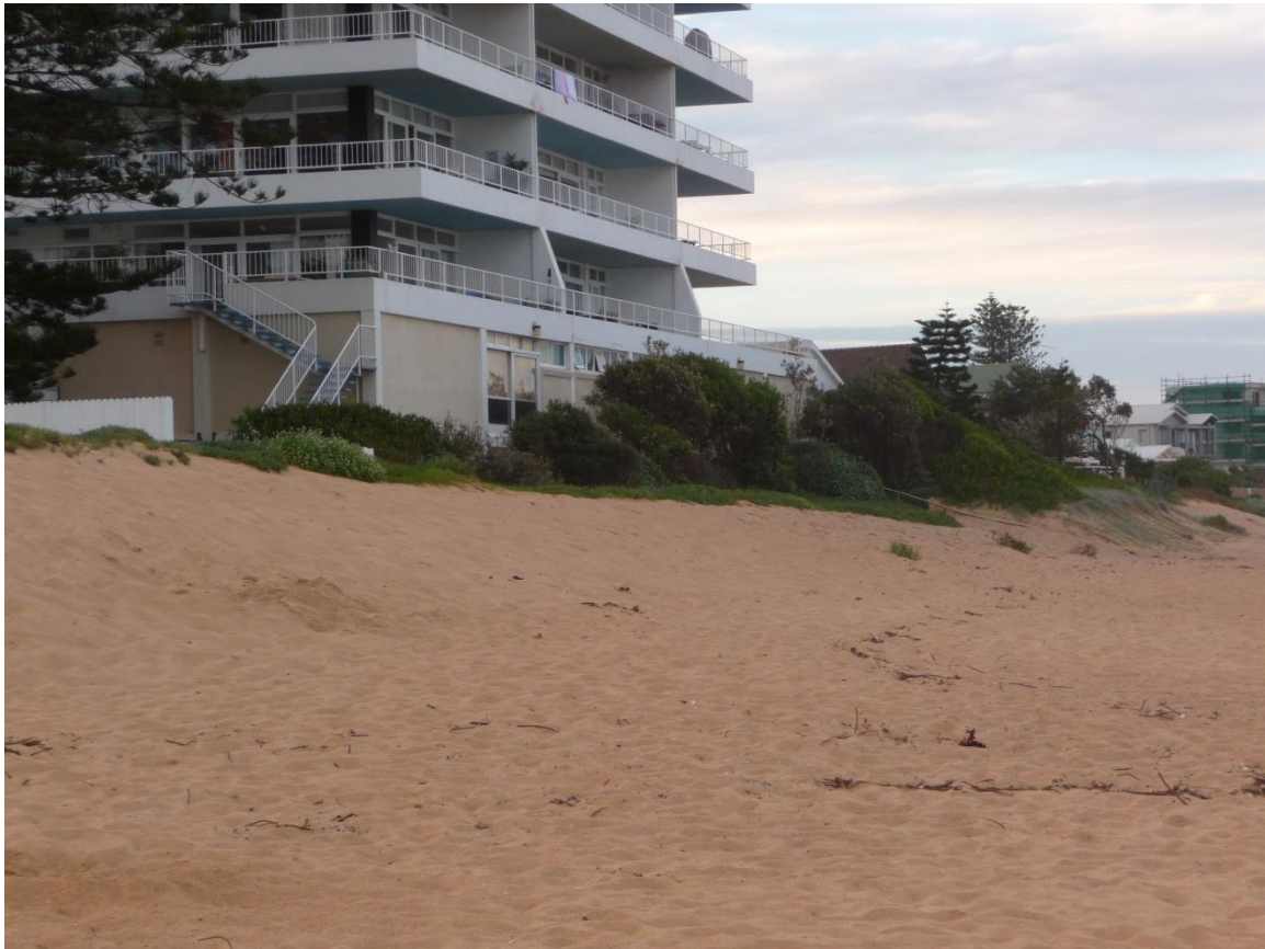
Figure 4: Rock seawall exposed at “Flight Deck” in the 1970’s after a major storm (top, courtesy of Don Champion), and (bottom) the same site in 2009, with the rock seawall buried under sand (typical conditions)
